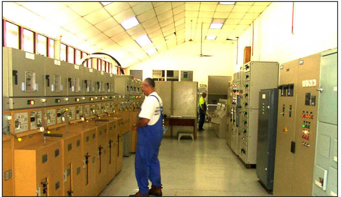
The Control Room
